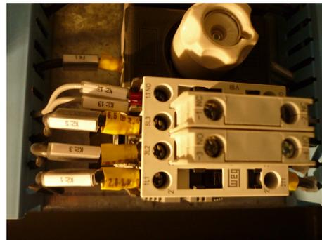
Figura 4.4: Contactor -  $I_n = 9A$
