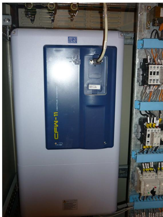
Figura 4.10: Módulo Conversor CFW11-105-RB
