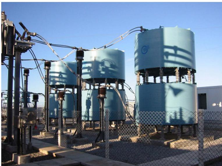
Figura 7 – Reator Controlado a Tiristor – TCR<sup>10</sup>
